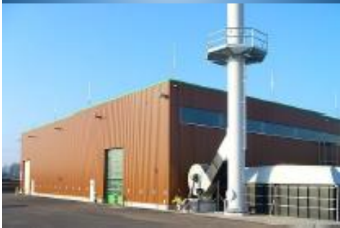
Mechanical Treatment Tailored RDF - System
